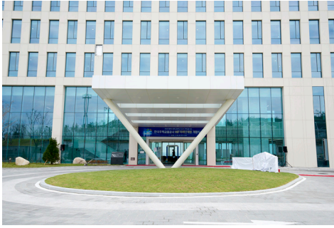
Exterior of HF Future Talent Center
